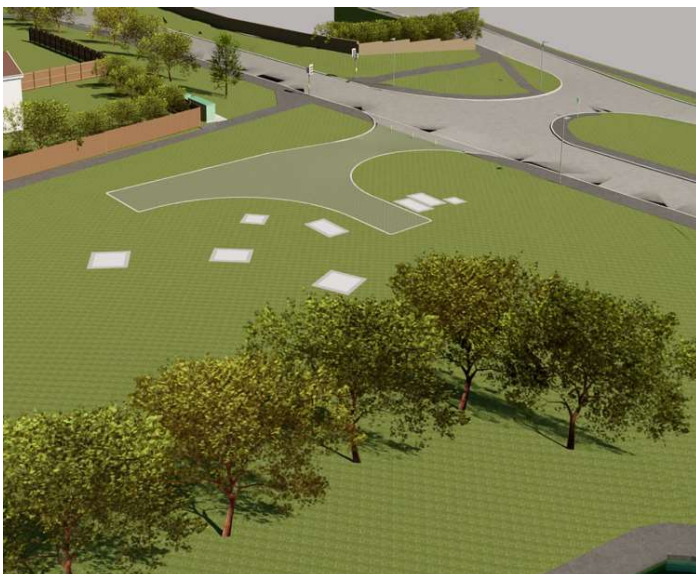
Post works artist impressions of how the tank area will look once works are completed. Only tank/chamber covers, grasscrete access road and control kiosks visible.
