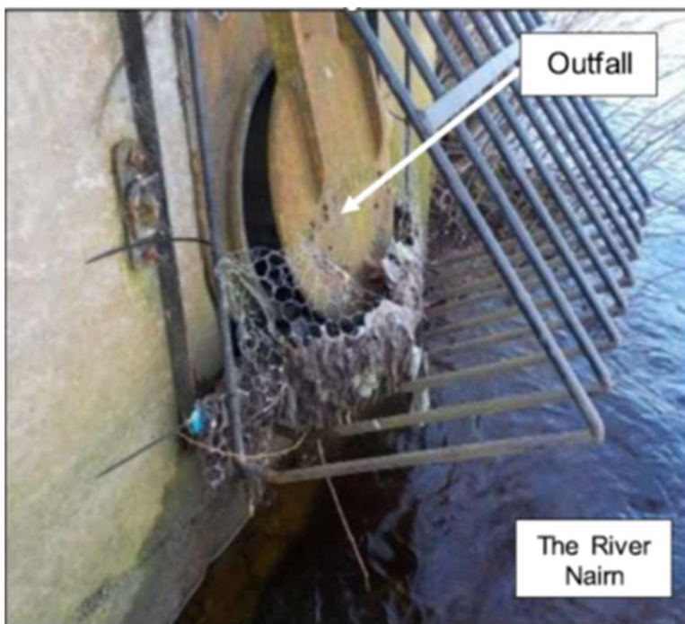
River Nairn Outfall
