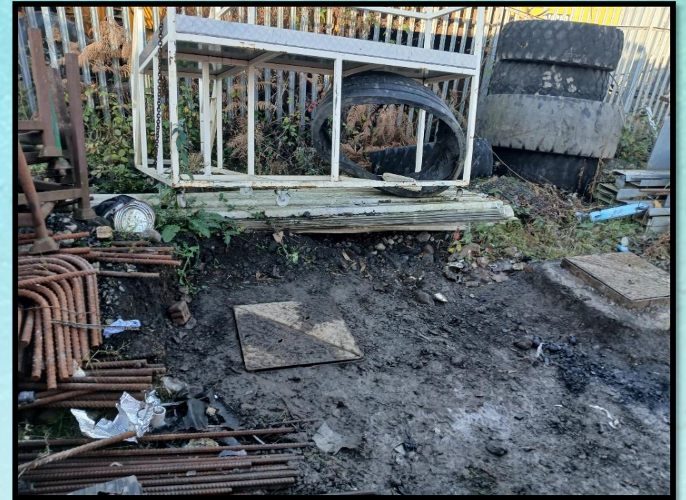
Existing Storm Overflow Chamber
