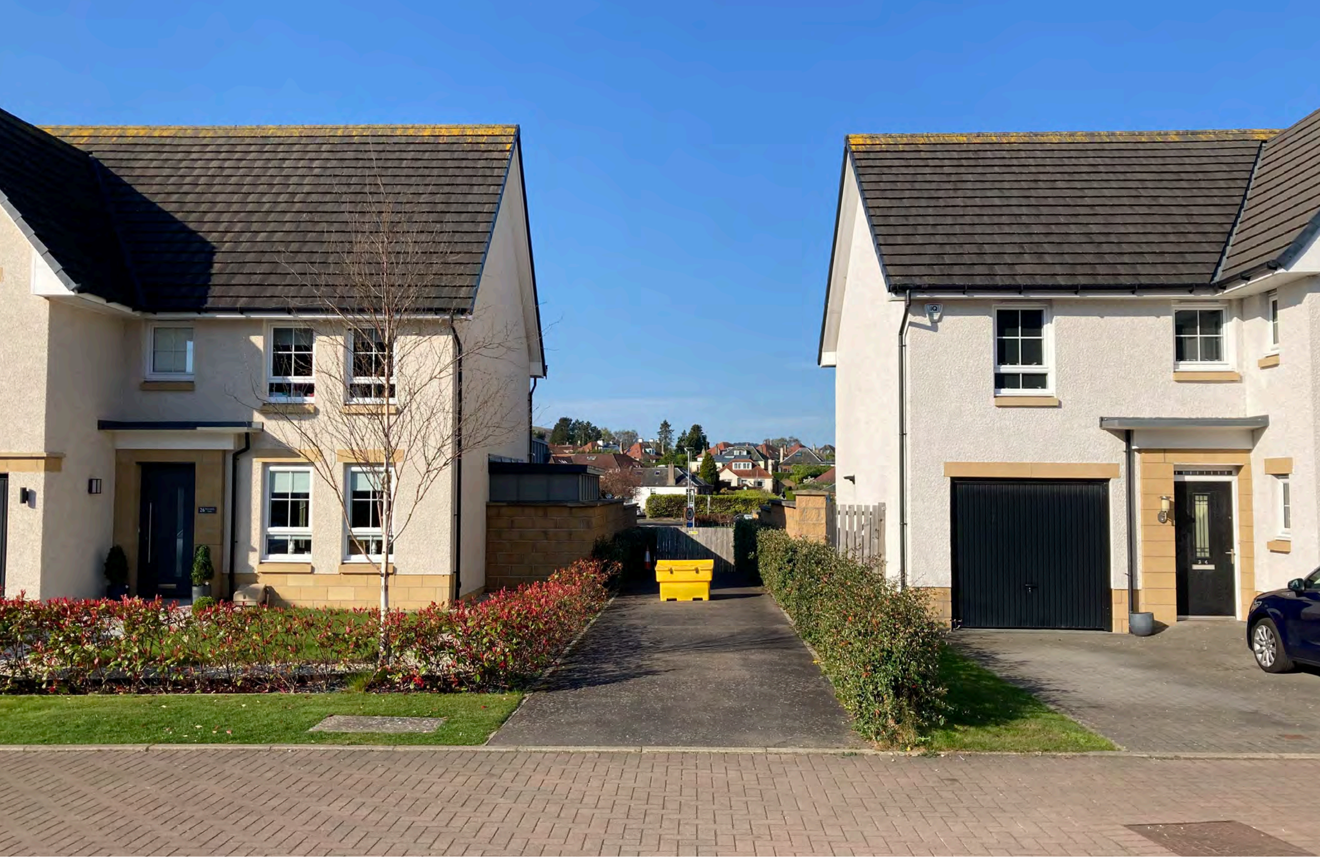
Existing path to north of the site from Skerryvore Loan, looking south
