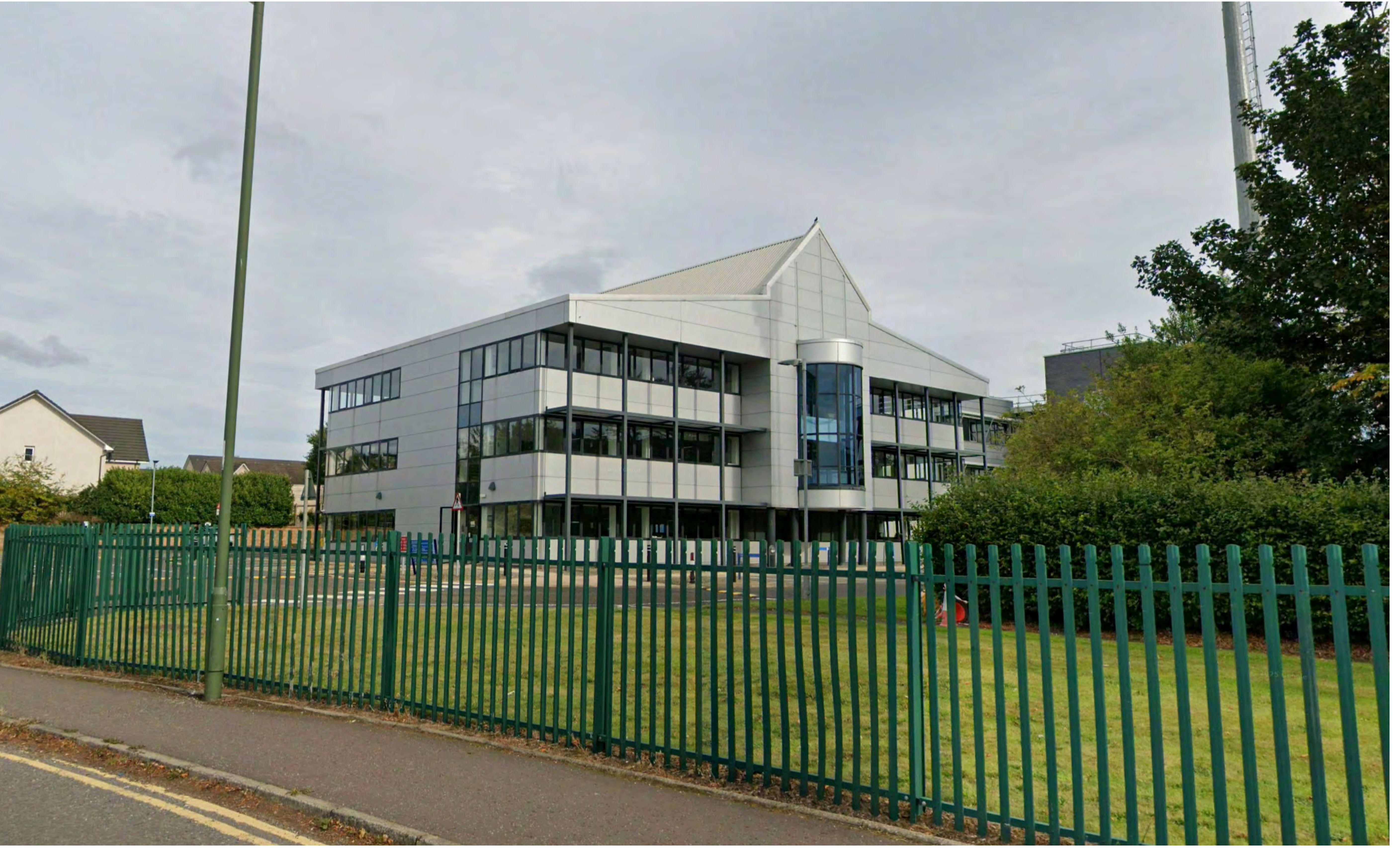
View into site from Waterfield Road.
