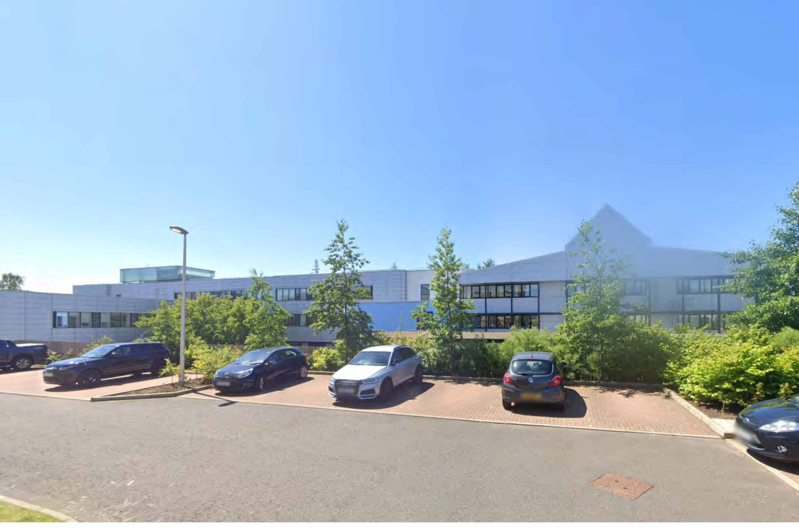
View of northern boundary from Fairfield Gardens.
