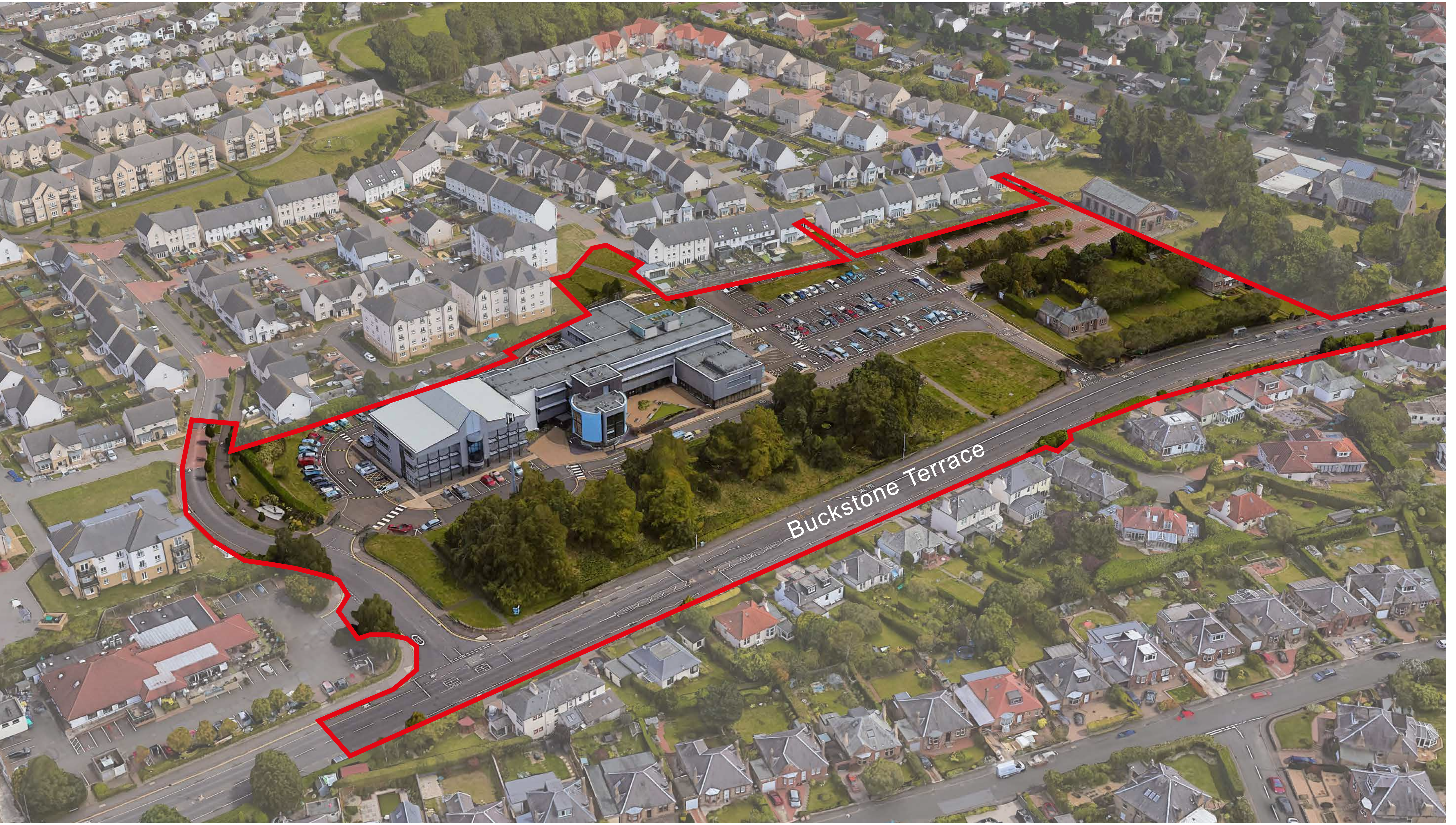
Aerial image of site looking east.
